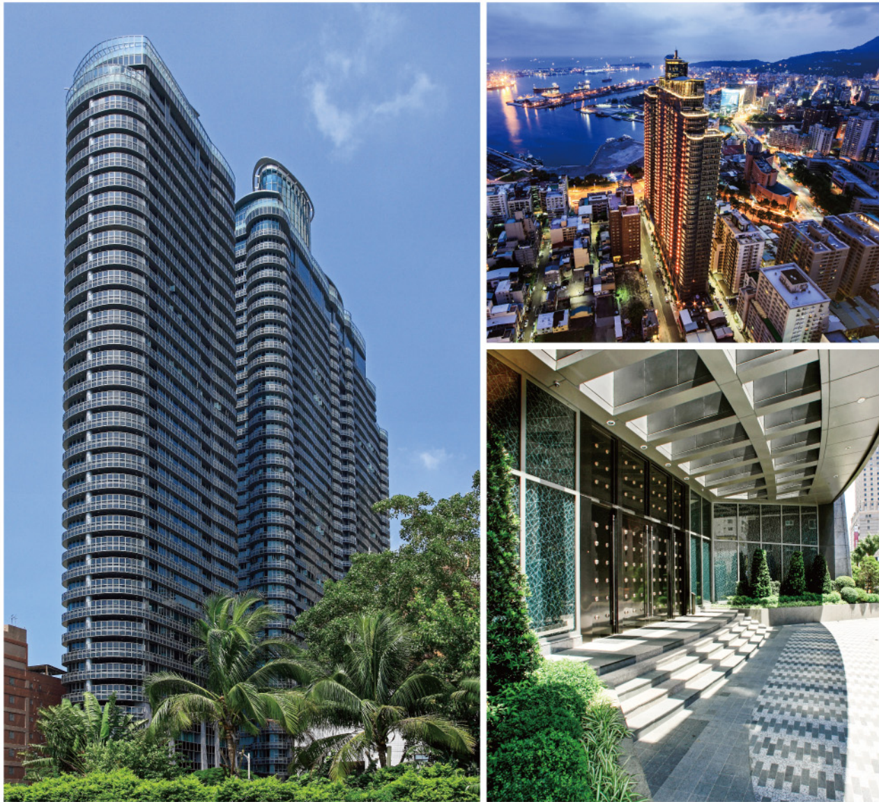
Project Name: Kuo Yang Kuo-Yan Condominium Client: Kuo Yang Construction Location: Kaohsiung City, Taiwan Duration: September 2010 to September 2013 Description: Constructed by CEC, the 41-story Kuo Yang Kuo-Yan Condominium is the tallest residential skyscraper in Taiwan. The building features an iconic yacht-shaped roof top, a 5-level basement and comprises three buildings with 82,527 m 2 of total floor area.
