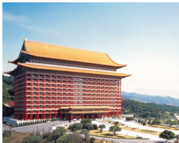
One of CEC's most recognized icons is the Chinese palace style Grand Hotel, completed in 1973.
