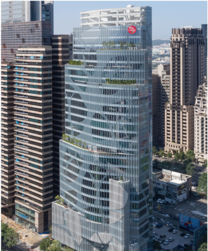
Project Name: CTBC Taichung HQ Client: Continental Development Corporation Location: Taichung City, Taiwan Duration: July 2015 to December 2017 Description: CEC undertook the China Trust Bank Corporation (CTBC) Taichung HQ construction project. Spanish architecture studio EMBT (designers of the Spanish Pavilion at Expo Shanghai 2010) designed the building, incorporating multiple-curtain wall design to form a huge pine tree to commemorate the late CTBC Holdings founder Jeffrey Koo Sr.’s passion for the brand’s spirit. The CTBC tagline “We are family”, is represented by numerous pine cones hanging from the tree’s branches. CTBC Taichung HQ is a 28-story office tower standing nearly 125 m tall.
