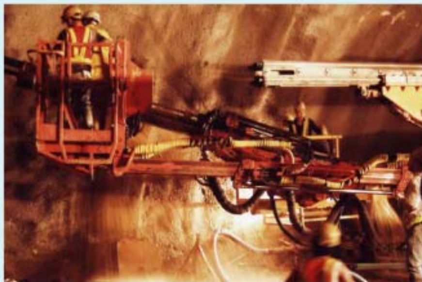
▲ Drilling works at Tunnel T3/6 T3/6 隧道黏孔
