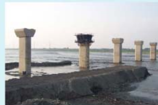
▲ C270 river crossing bridge C270標跨越河川橋樑
