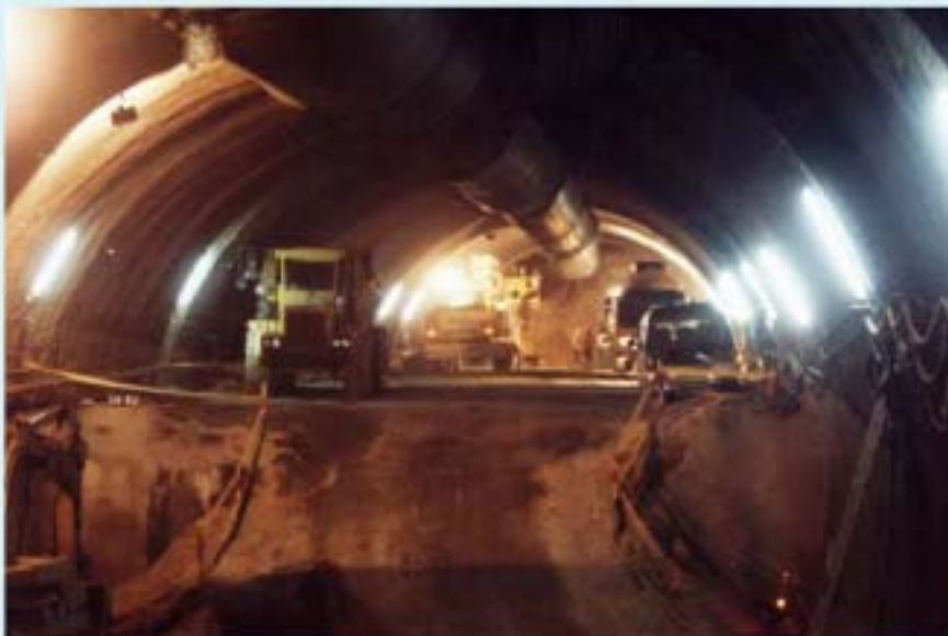
▲ Bench and heading at Tunnel T3/2 T3/2 隧道頂拱及平台開挖
