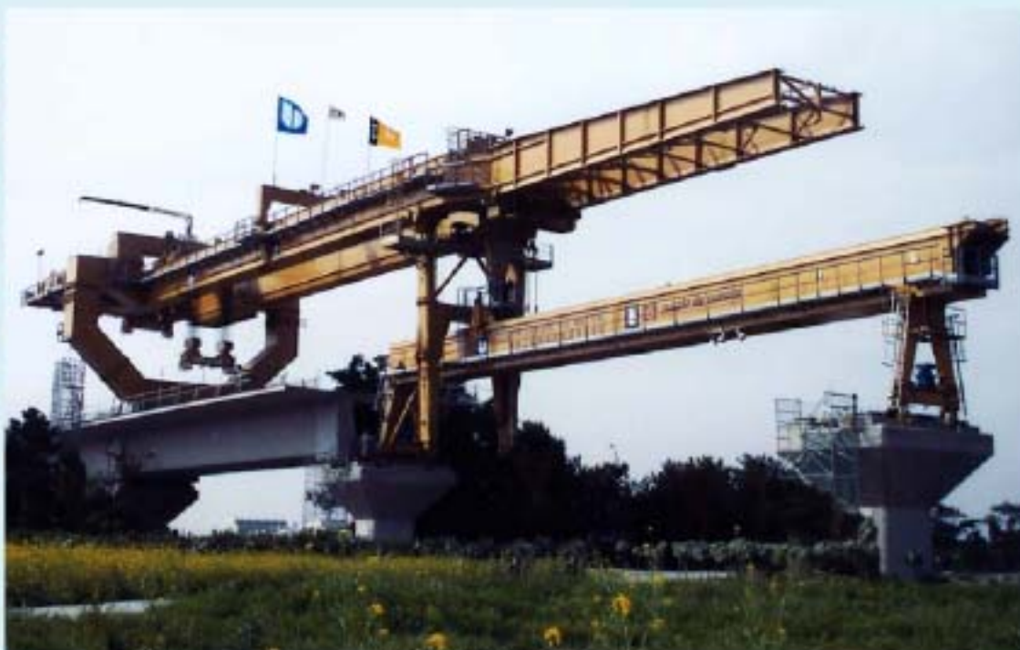
▲ Pre-cast span launching equipment 預鑄箱型梁吊裝設備
