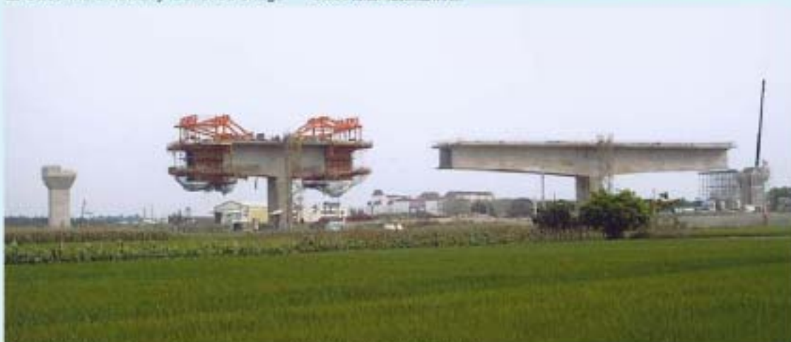
▲ C270 Balanced cantilever bridge C270標平衡懸臂工法橋樑
