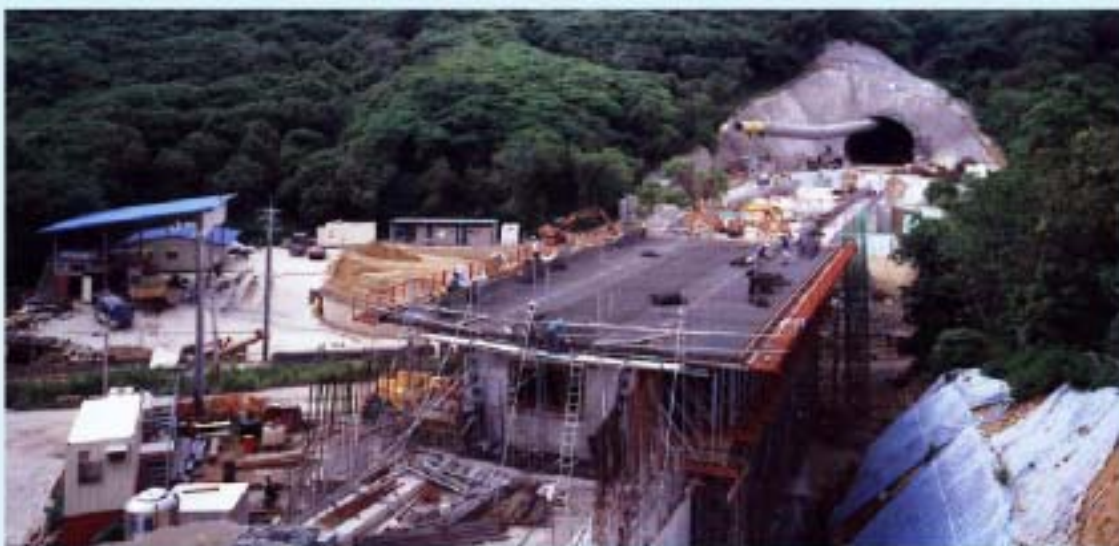
▲ C260 non standard bridge, earthworks and tunnel portal C260標非制式橋、路工及1號隧道南洞口
