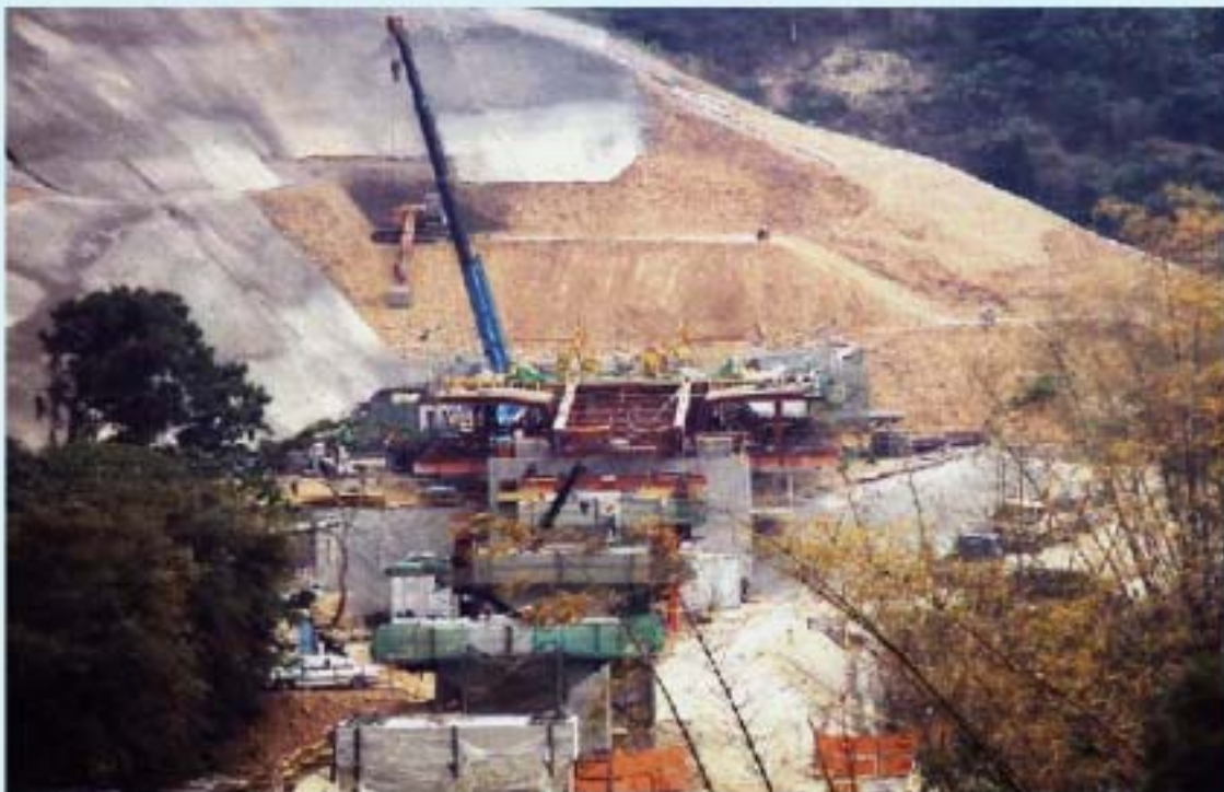
▲ C260 Incrementally launched bridge C260標節塊推進橋樑
