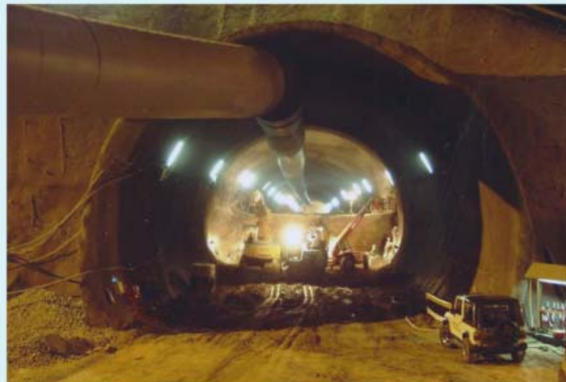
▲ Break through at Tunnel T1 T1 隧道貫通
