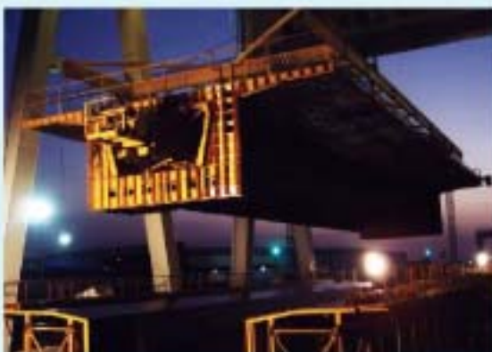
▲ Pre-cast span moulds in operation 內模及預組鋼筋籠吊運
